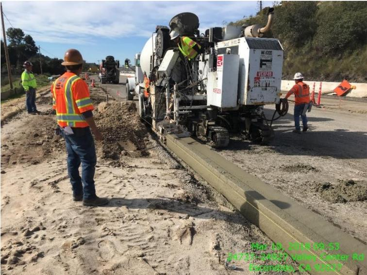
Figure 5. Placement of Curb and Gutter
