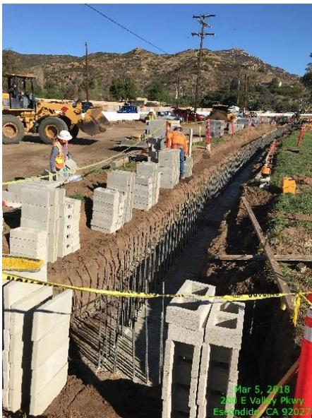
Figure 2. Eastern Sound Wall Foundation
