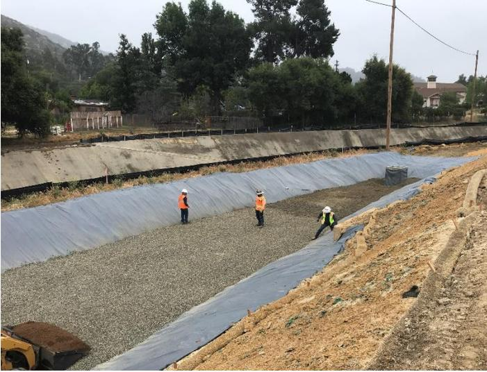
*Figure 4. Construction of bio retention basin*
