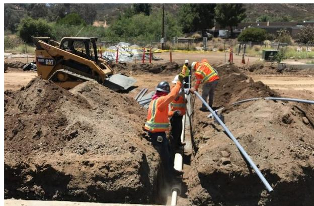
*Figure 3. Installation of irrigation services*
