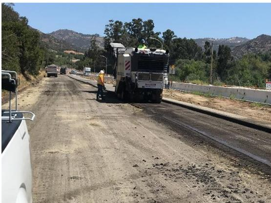
*Figure 2. Grinding of the old asphalt roadway*
