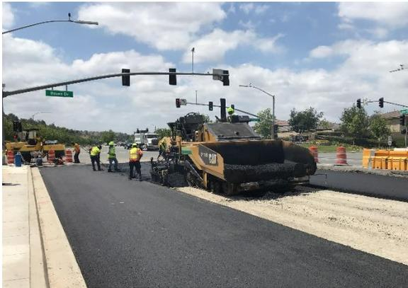
*Figure 1. Asphalt base pave operation*
