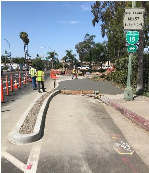
Figure 3. Bike Path Transition at New Driveway
